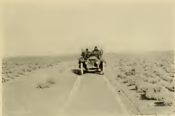
It would be difficult to find an equal continuous mileage of good natural gravel road as that reaching across the State of Nevada from Ely to Tonopah
